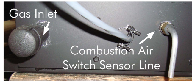
Figure 17a. Identifying the Gas Inlet and Combustion Air Switch Sensor Line
