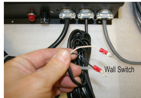
Figure 15c. (Remote Switch Wire connection)
