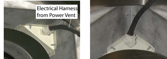
Figure 11e. Installed power harness.
